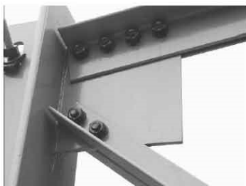
Figure 7-17. Misc. Connection: Truss Column C2 / Truss B7
